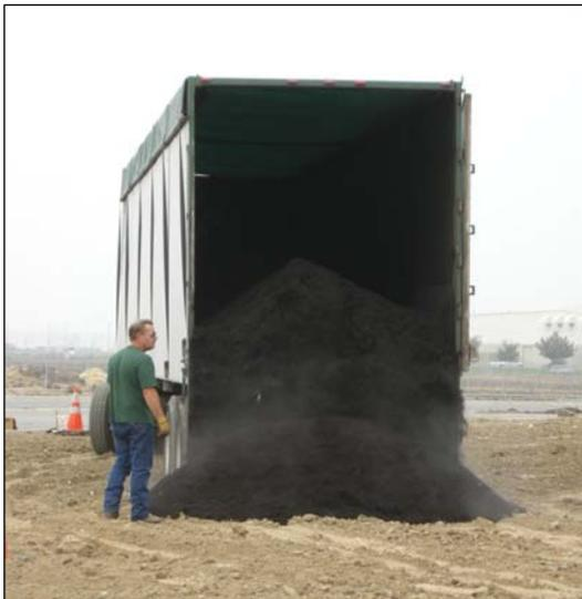
**Figure 3. Twenty-three tons of compost/ gypsum added to 13,000 sq. ft. future garden site.**
